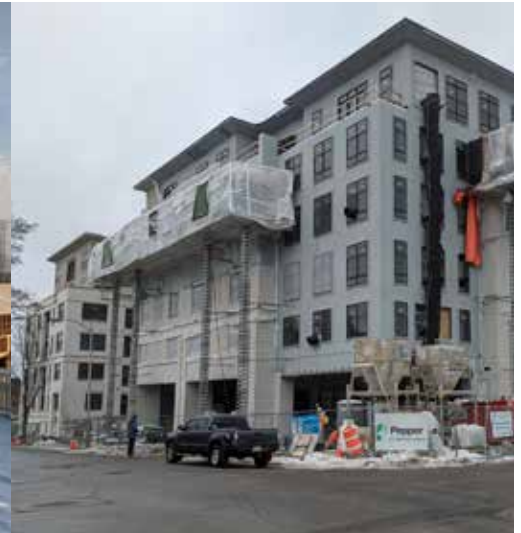
Left: Back courtyard view of Grace Commons which will include a bocce court, seating, and walking paths. Right: Front entrance of St. Rita Square into the lobby and trattoria.
